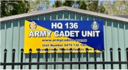
New renovations of HQ 136 ACU.
